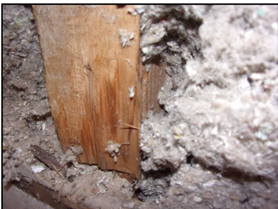
65: Typical wood framing element in Town Hall
