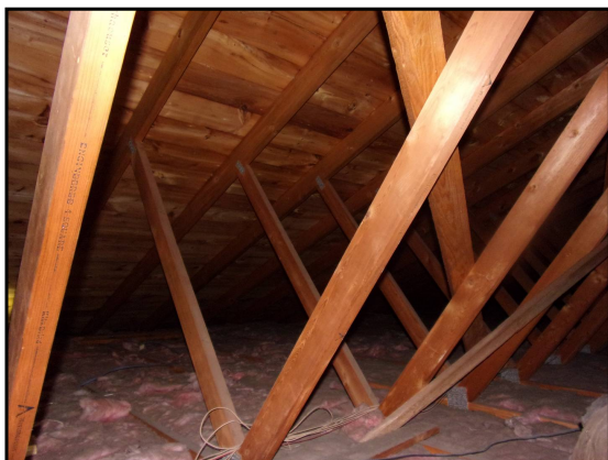
77: Fire House attic framing
