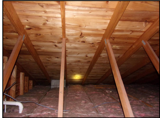
74: Fire House attic
