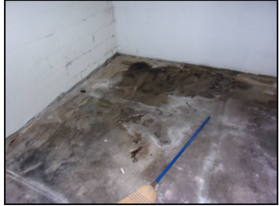
68: Fire House concrete floor slab
