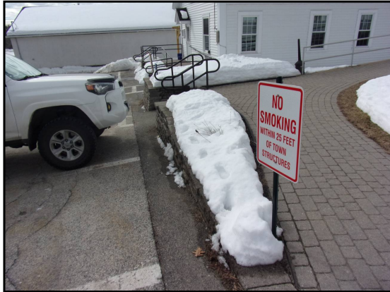
25: Exterior walk with concrete pavers
