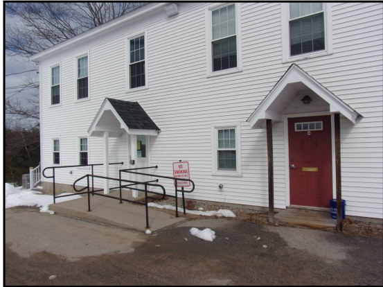
13: South side of Admin Offices
