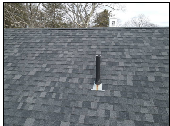
36: Admin Office roof with vent
