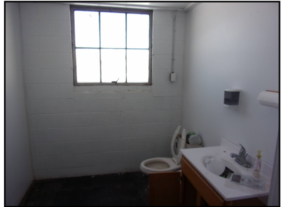
70: Restroom in Fire House
