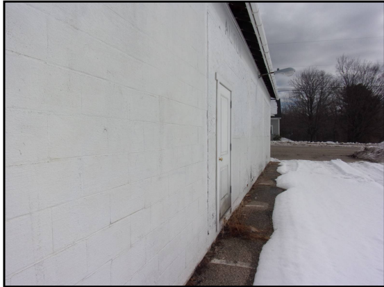
19: South side of Fire House
