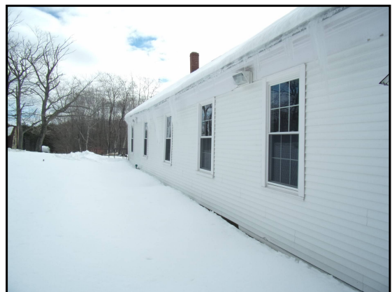
6: North side of Town Hall
