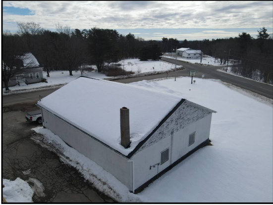
37: Aerial view of Fire House
