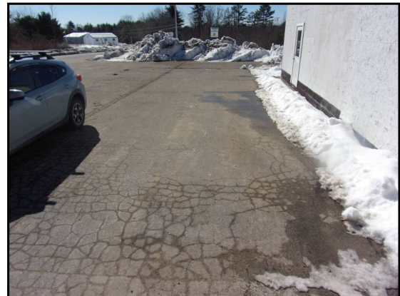
28: Pavement along north side of Fire House
