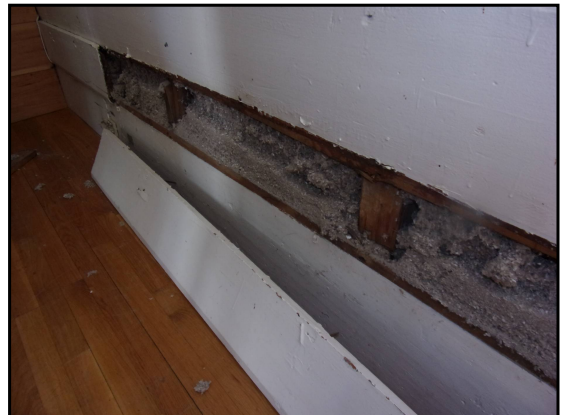
64: Exposed wood framing in Town Hall
