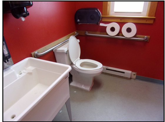
46: Public restroom in Admin Office / Town Hall
