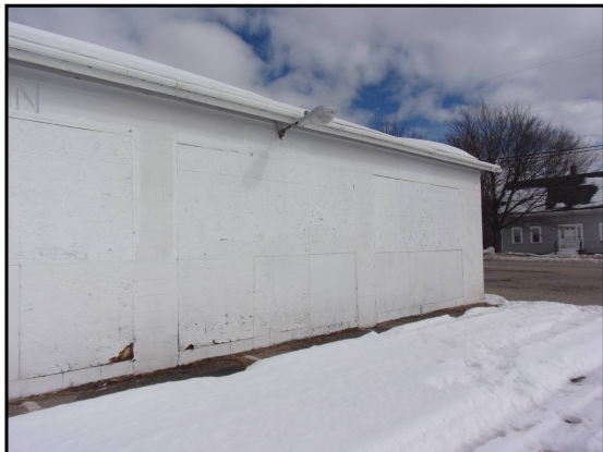
21: South side of Fire House with truck bays
