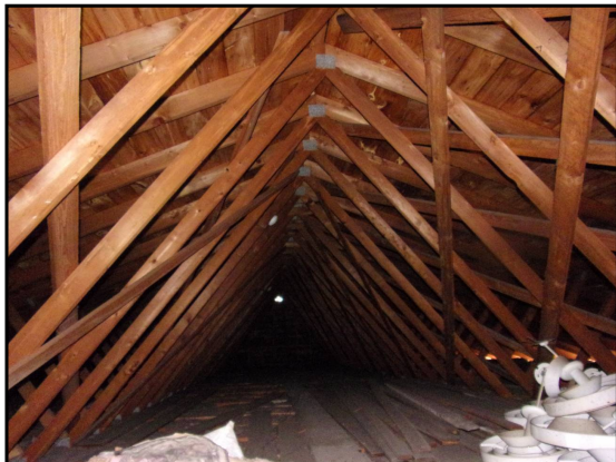
75: Fire House attic
