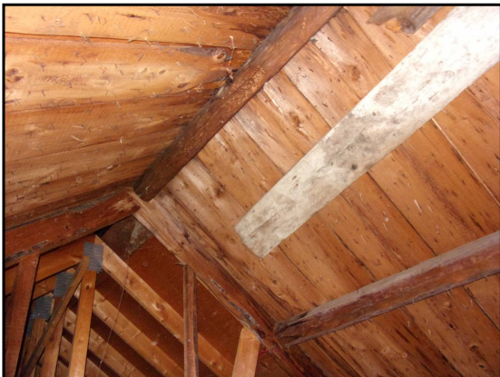
63: Town Hall roof decking and framing
