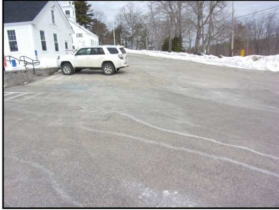
31: General asphalt condition
