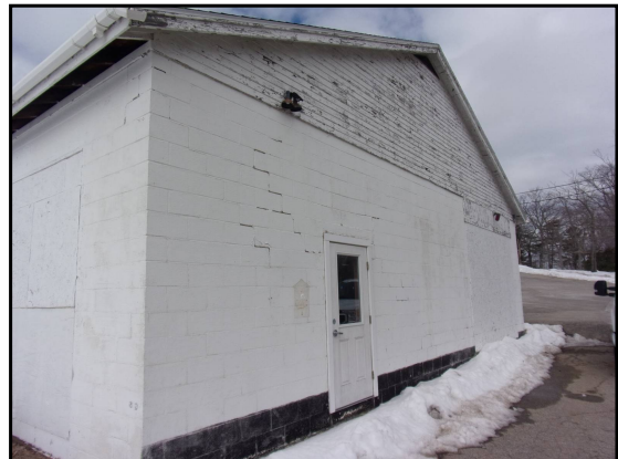
22: East side of Fire House
