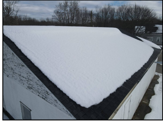
38: Fire House roof
