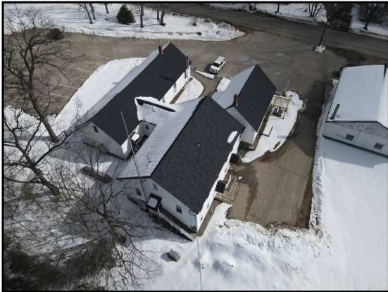
39: Aerial view from the west
