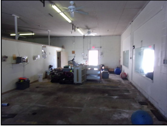
67: Interior of Fire House
