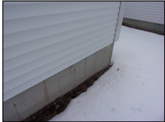
10: Foundation wall of Admin Offices
