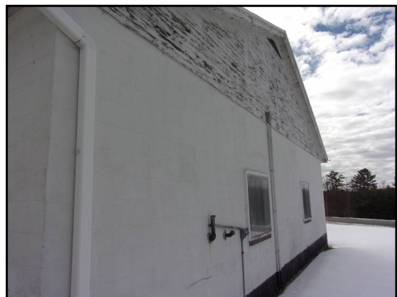
18: West side of Fire House
