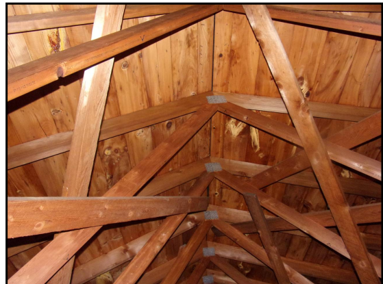
76: Fire House attic framing and roof deck
