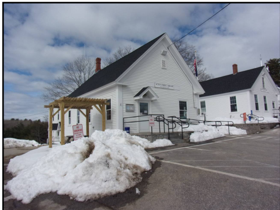
15: View of Library and Town Hall
