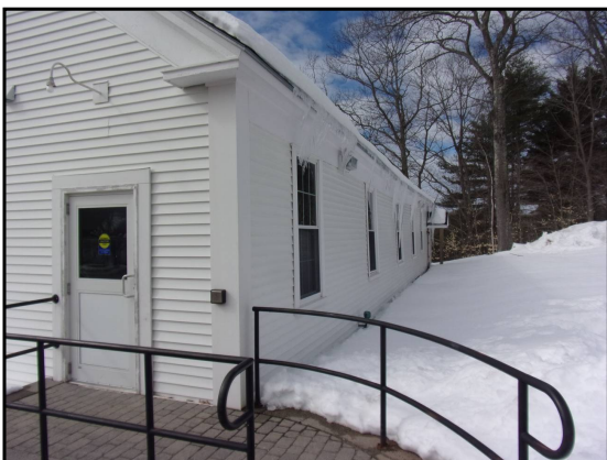
5: Entry ramp with pavers and metal handrails
